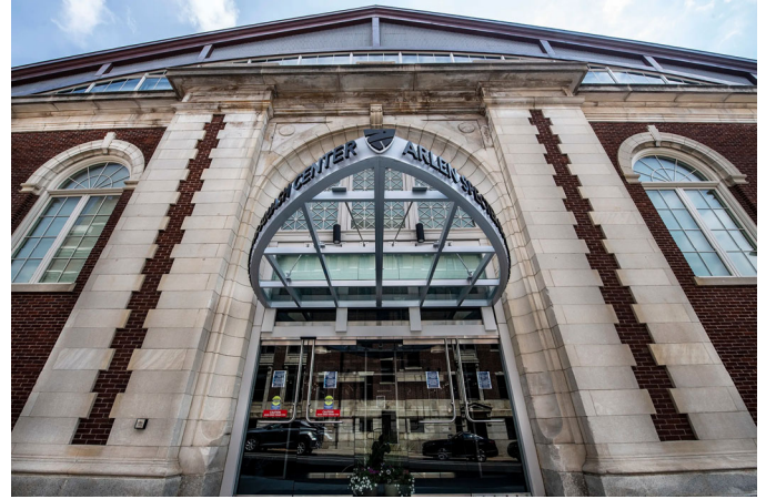
After acquiring the historic armory from the state, Drexel University completely renovated the Classical Revival facade and restored the windows, which had been bricked up. The building is now the home of the US Squash's Specter Center
